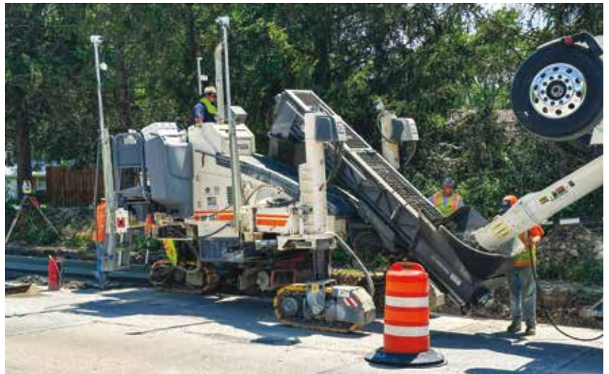
Kinney Contractors uses a WIRTGEN SP 15i offset slipform paver with WIRTGEN AutoPilot 2.0 on a curb project.
