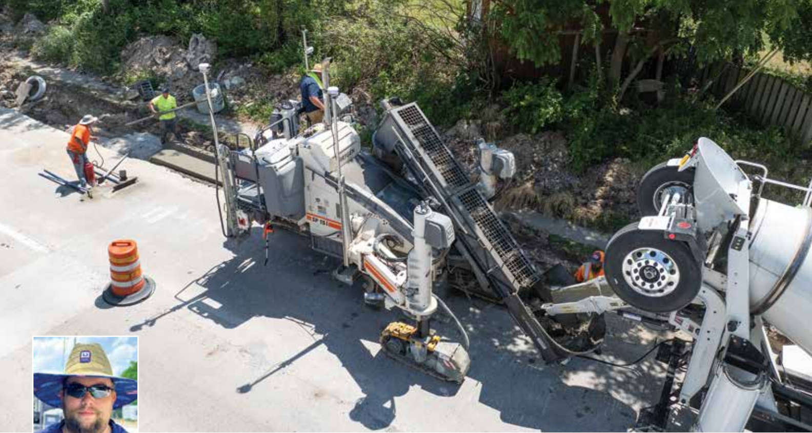
Kinney Contractors utilizes a WIRTGEN SP 15i offset slipform paver that features WIRTGEN AutoPilot 2.0. "I believe Kyle McDowell and Roland's help was a big factor in our ability to add the machine and have success with it," said operator J.D. Moore.
